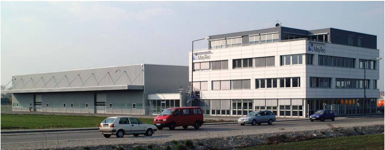
MayTec GmbH plant in Dachau
